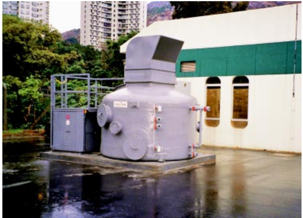
Pumping station located in city center
