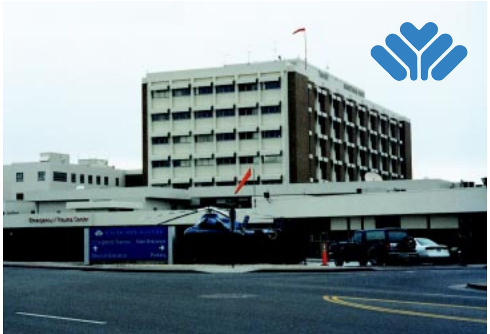
Washoe Medical Center - Main Building
