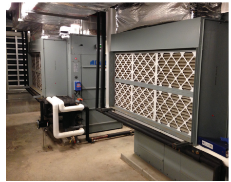
DRY-O-TRON® DSV-080s w/Chloraguard® filter racks relocated in the wall to protect entire mechanical room.
