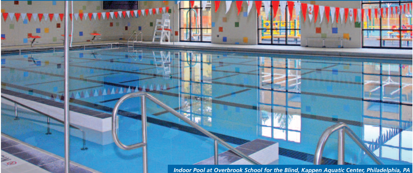
Indoor Pool at Overbrook School for the Blind, Kappen Aquatic Center, Philadelphia, PA
